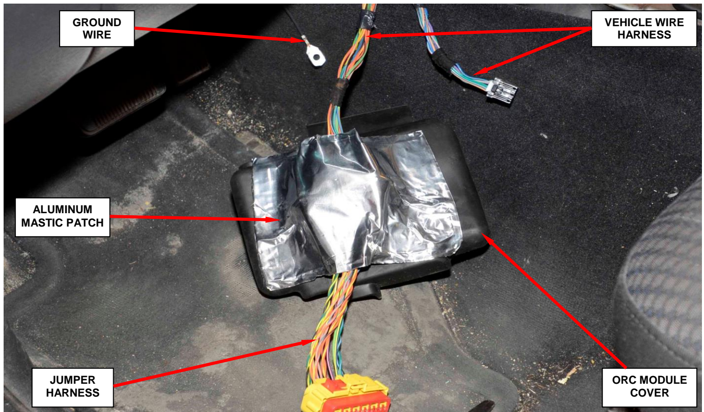
Figure 10 – Install Aluminum Mastic Patch
